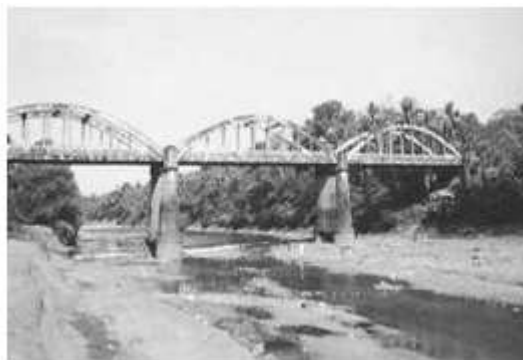
Fig01- River bank erosion in Oha oya River
