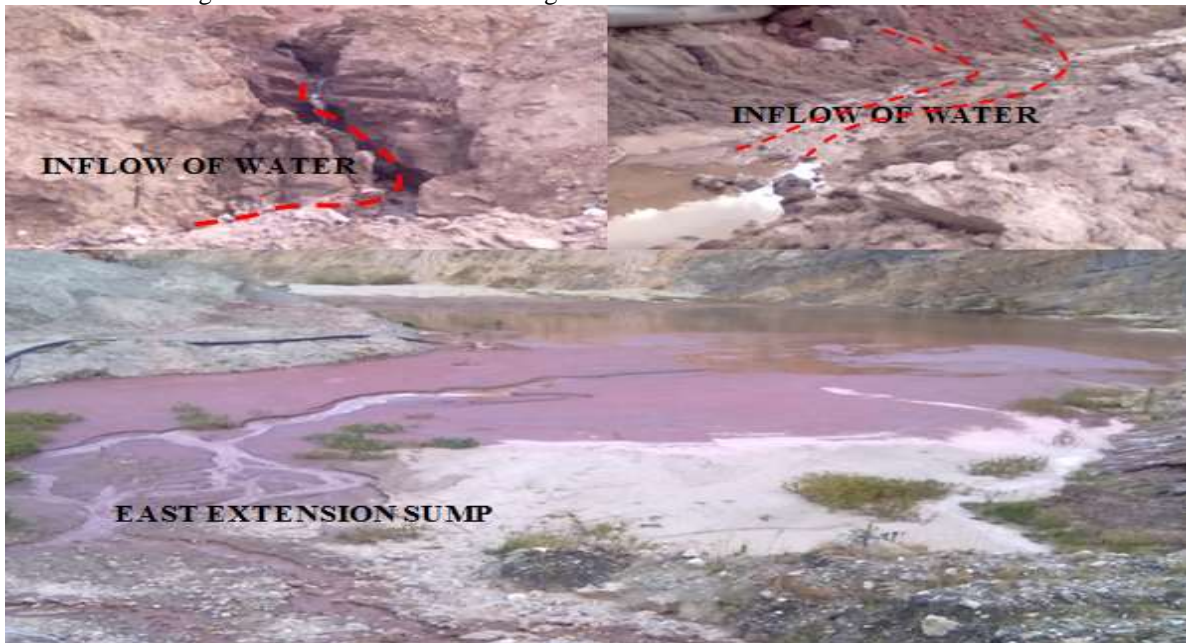
Figure 10: Sub - surface water percolating through the NOP Foot wall slopes (top) and the Eastern Extension sump
